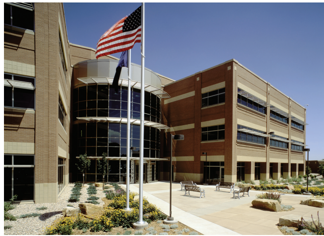
The Centre for Advanced Technology in Fort Collins features several Everitt Commercial Partners-managed projects including the recently completed Natural Resources Research Center pictured above.
